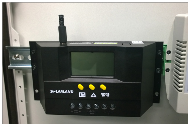
Thermal Sensor Plugged into Controller
