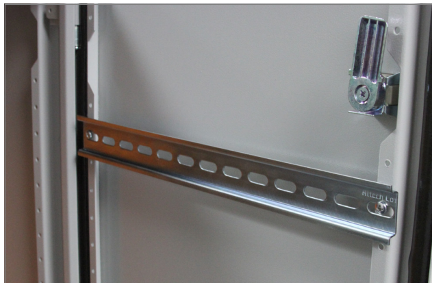
DIN Rail installed on door
