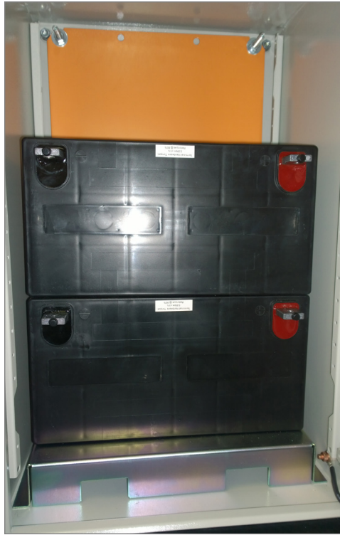
Batteries Placed into the Enclosure
