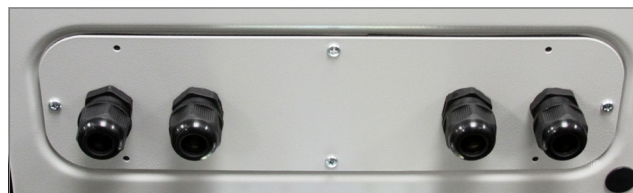
Battery Platform on Floor of Enclosure
