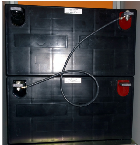
PV Cable Connecting Battery Terminals
