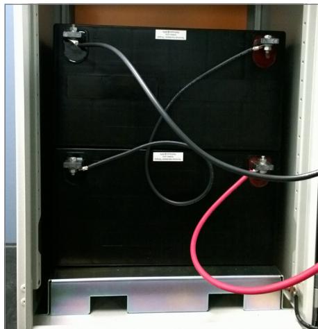
PV Cable Connecting Battery Terminals
