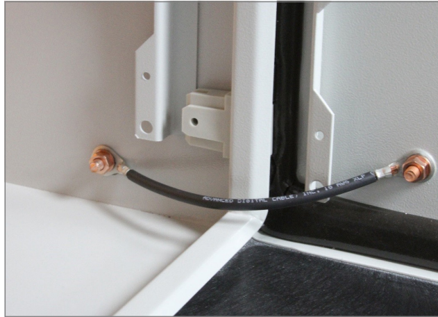
Grounding Cable Installed
