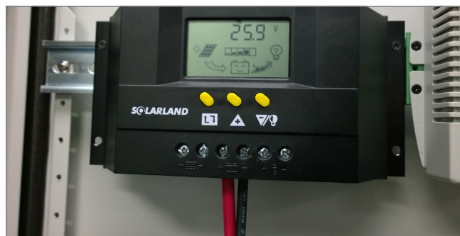
Battery Cables Connected to Controller Battery Terminals
