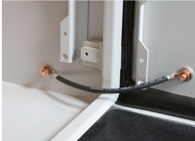
Grounding Cable Installed
