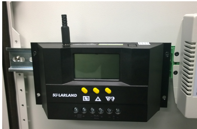
Thermal Sensor Plugged into Controller
