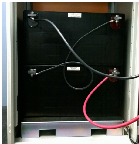
PV Cable Connecting Battery Terminals
