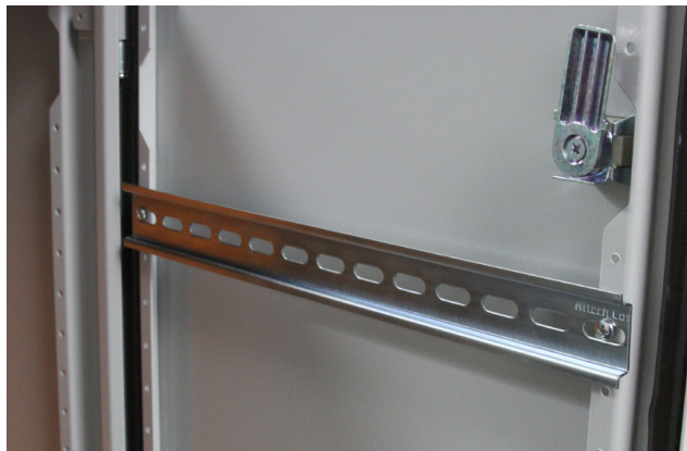
DIN Rail installed on door
