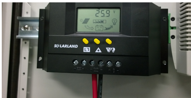
Battery Cables Connected to Controller Battery Terminals
