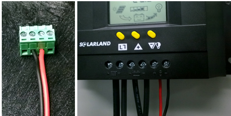
Red and Black Cable Connected Green Terminal Connector, left, and to Load Terminals on Controller, right.
