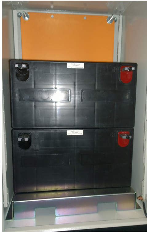
Enclosure Mounted to Pole with Clamps
