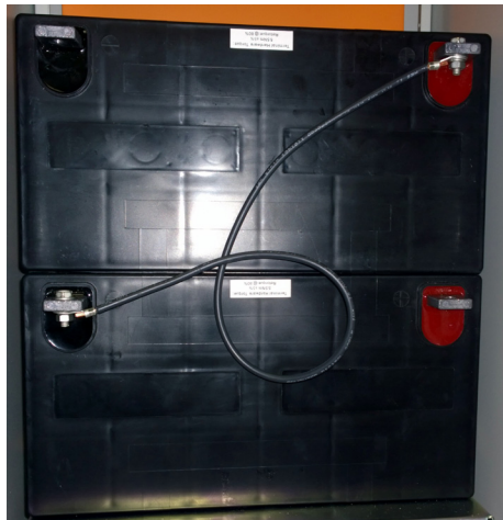
PV Cable Connecting Battery Terminals
